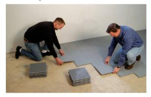
Basement Systems solution is a ThermalDry Basement Floor Matting system. This consists of a specially engineered polypropylene, 12-inch tongue-&groove square tile that, unlike systems that use wood, is totally water and vapor proof. The unique grid design on the bottom of the tile creates an air space that insulates the floor, and does not cause water vapor to condense. The installation takes away only ¼" of precious ceiling height in the basement, instead of 4" for other methods.
