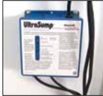
The UltraSump® includes its own DC-operated pump, a second automatic-switching system, a 'smart' charging system, and a specially-designed battery.
