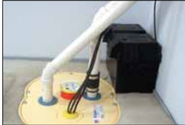
The UltraSump® includes its own DC-operated pump, a second automatic-switching system, a 'smart' charging system, and a specially-designed battery.
